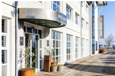
Pier 5 Hotel Aalborg
